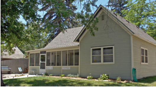
Front of building
